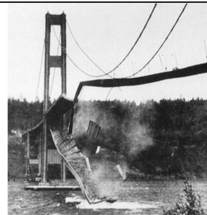
Tacoma Narrows Bridge on the morning of Nov. 7, 1940. The bridge was an unusually light design, and, as engineers discovered, peculiarly sensitive to high winds. Rather than resist them, as most bridges do, the Tacoma Narrows tended to sway and vibrate. On November 7, in a 40-mile-per-hour wind, the center span began to sway, then twist. The combined force of the winds and internal stress was too great for the bridge, and it self-destructed. No one was killed, as the bridge had been closed because of previous swaying. This is one of the best-known and most closely studied engineering failures, thanks in large part to the film and photographs that recorded the collapse.
