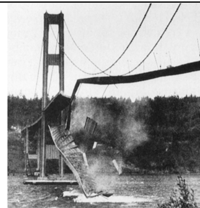
Tacoma Narrows Bridge on the morning of Nov. 7, 1940. The bridge was an unusually light design, and, as engineers discovered, peculiarly sensitive to high winds. Rather than resist them, as most bridges do, the Tacoma Narrows tended to sway and vibrate. On November 7, in a 40-mile-per-hour wind, the center span began to sway, then twist. The combined force of the winds and internal stress was too great for the bridge, and it self-destructed. No one was killed, as the bridge had been closed because of previous swaying. This is one of the best-known and most closely studied engineering failures, thanks in large part to the film and photographs that recorded the collapse.
